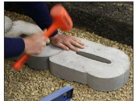
Diagram 3—Lay and level base block
