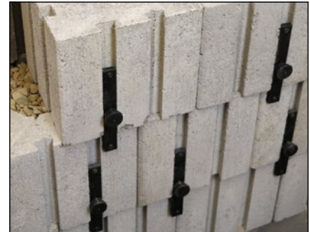
Diagram 6—Lock connector to the block in front
