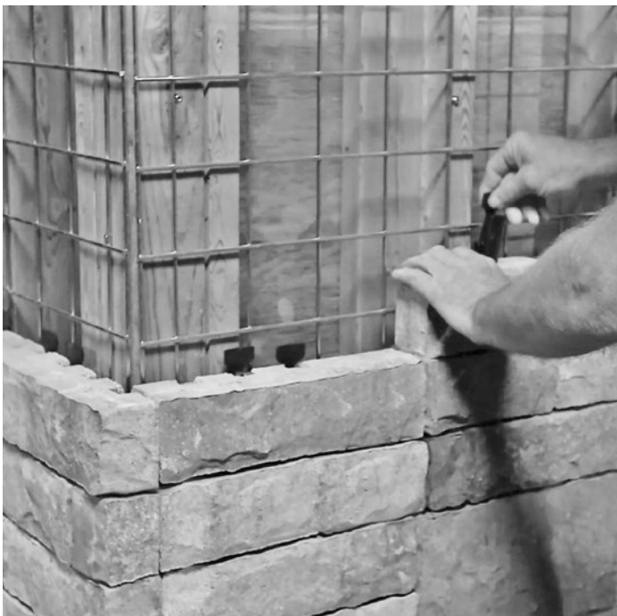
Attach Lafitt Tandem Veneer with Connector
