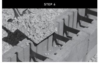
Place 3/4" crushed rock in between the panels to provide frictional connection and proper internal drainage.
