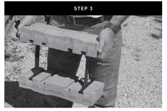
Assemble the Tandem Wall units by inserting the Tandem Wall connectors into the dove tails. Make sure the front and rear panels are the same length.
