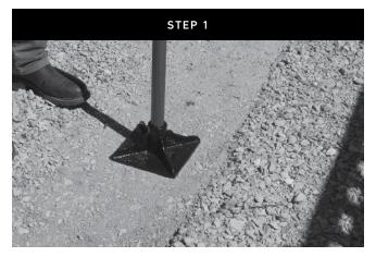
Remove all surface vegetation and debris. Select the length of the wall and excavate a trench the length of the wall and approximately 12" from top of final grade. Then place a minimum of 6" of dense graded aggregate and compact to 95% standard density or modified. It's not recommended to use a pea rock or a rounded type of material on the base.
