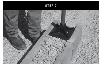
Lightly hand compact the gravel in between the panels for proper compaction.
