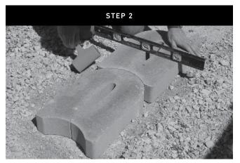
Place the Base Block (shown here) on the compacted gravel. Level the base block units front to back as well as side to side. Making sure the units are fully level.
