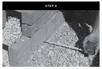
Place 12" of 3/4" drainage rock behind the rear panel of the wall. This will provide for proper drainage behind retaining walls.
