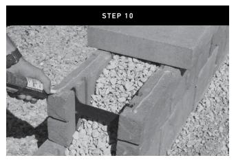
When placing the cap on top of Tandem Wall, use a construction adhesive to secure the cap to the top of the wall.
