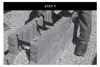
Set additional courses of the Tandem Wall. Making sure that you are keeping the wall in proper alignment. Backfill and compact each additional course.
