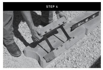
Place the assembled Tandem Wall unit on the top of the U Start Base Block or Torpedo Base Block, making sure that the first course is centered on the base block. Check to make sure units are kept level.
