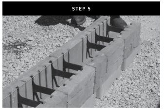
Once the Tandem Wall units have been placed. Run a string line along the back of the front or rear panel to assure you are keeping the wall units straight in line.
