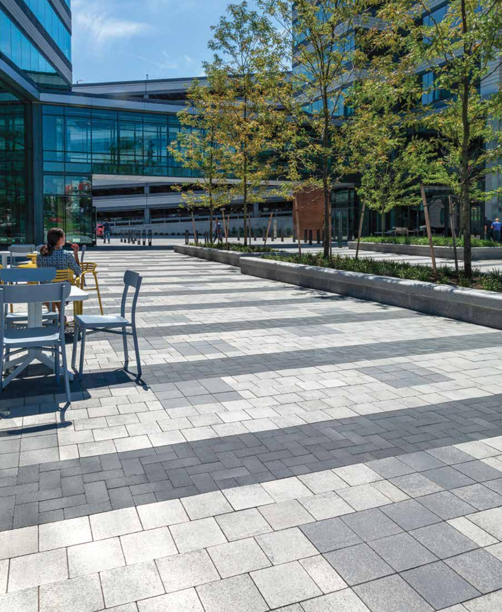
PROJECT: City Point, Waltham, MA. DESIGN: CBA Landscape Architects LLC. PRODUCT: 4 x 8" with Umbriano® finish in Midnight Sky and 8 x 8" with Umbriano® finish in French Grey and Grenada White.
