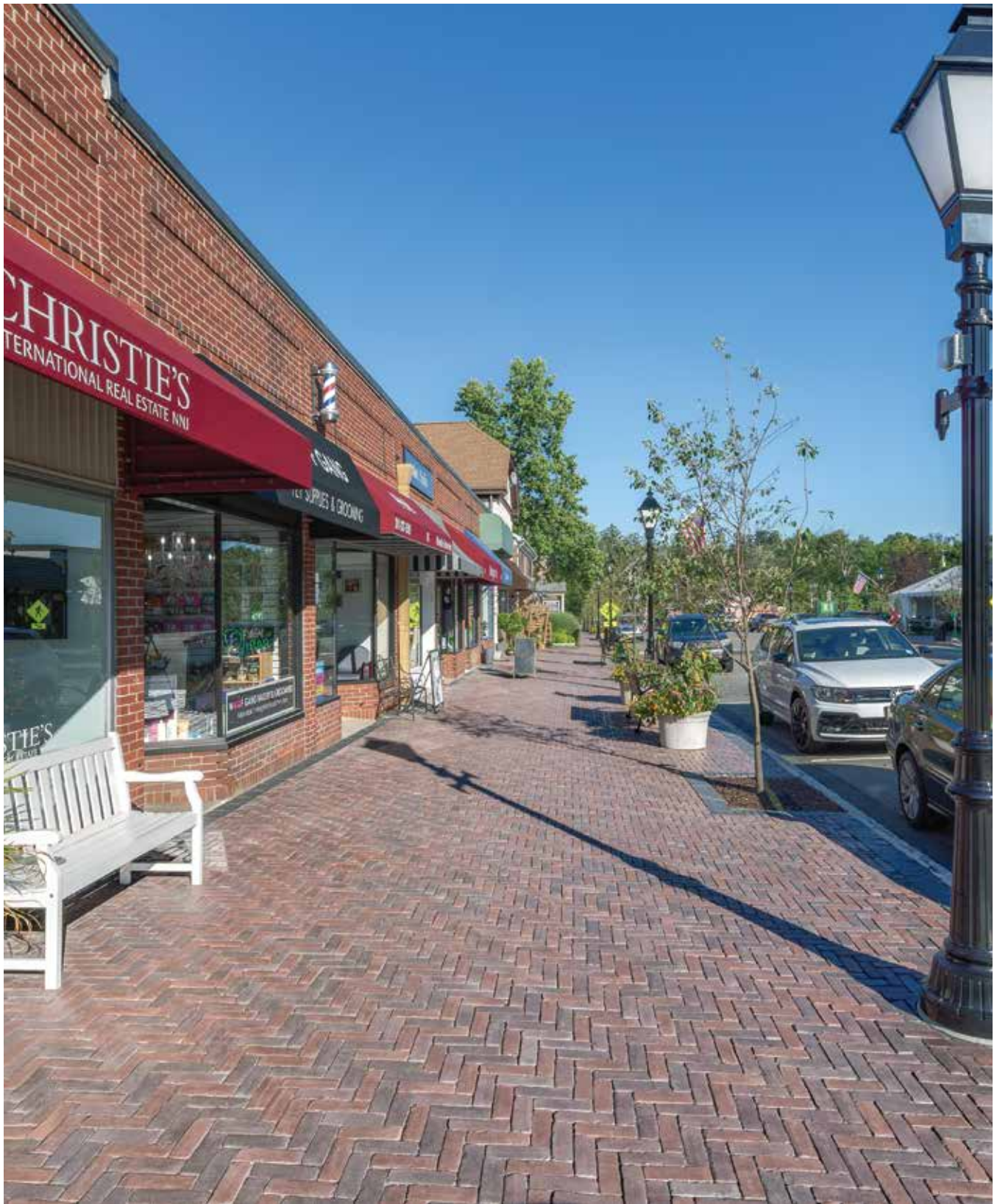
PROJECT: Allendale Streetscape, Allendale, NJ. DESIGN: Neglia - Engineering Associates. PRODUCT: Cophorne® in Burgundy Red, Burnt Clay, Old Oak, and Basalt.
