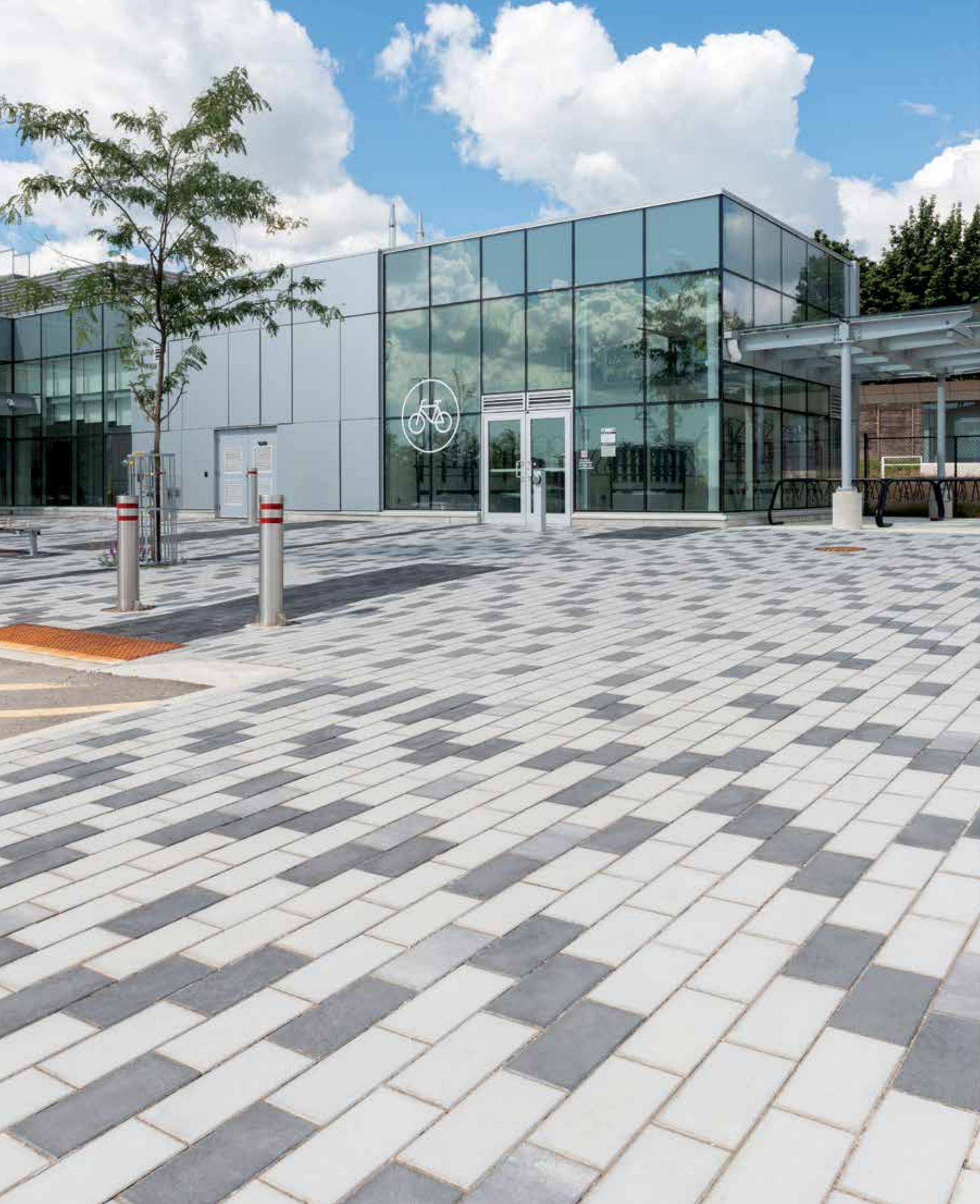
PROJECT: Cooksville GO Station, Mississauga, ON DESIGN: Brodies & Associates. PRODUCT: 7 x 14" with Smooth Premier finish in Granite Fusion, Midnight Charcoal and Opal Blend.
