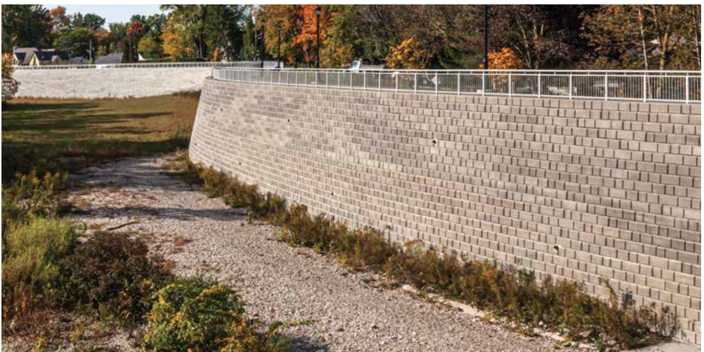
PROJECT: West London Dyke, London, ON. DESIGN: RisiStone Engineering. PRODUCT: DuraHold® in Natural.
