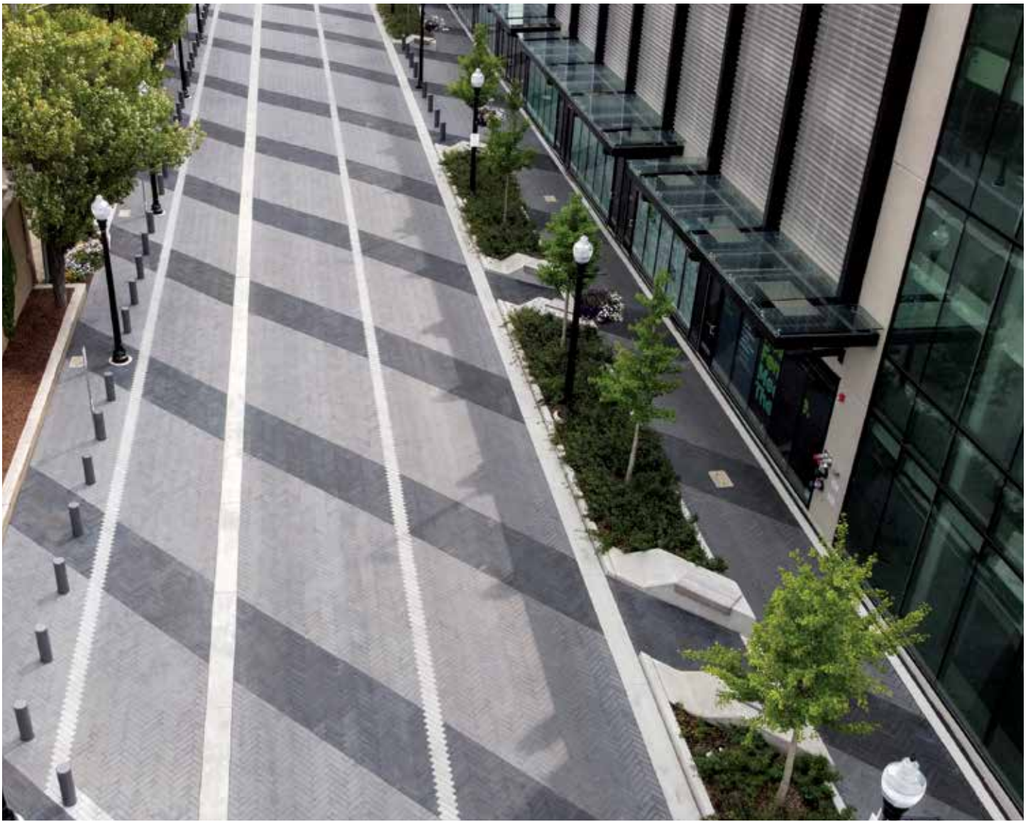
PROJECT: The DOT, Ferndale, MI. DESIGN: Grissim Metz Andriese Associates | Kenneth Weikal Landscape Architecture. PRODUCT: 4 x 16" with Smooth Premier and Series™ finishes.
