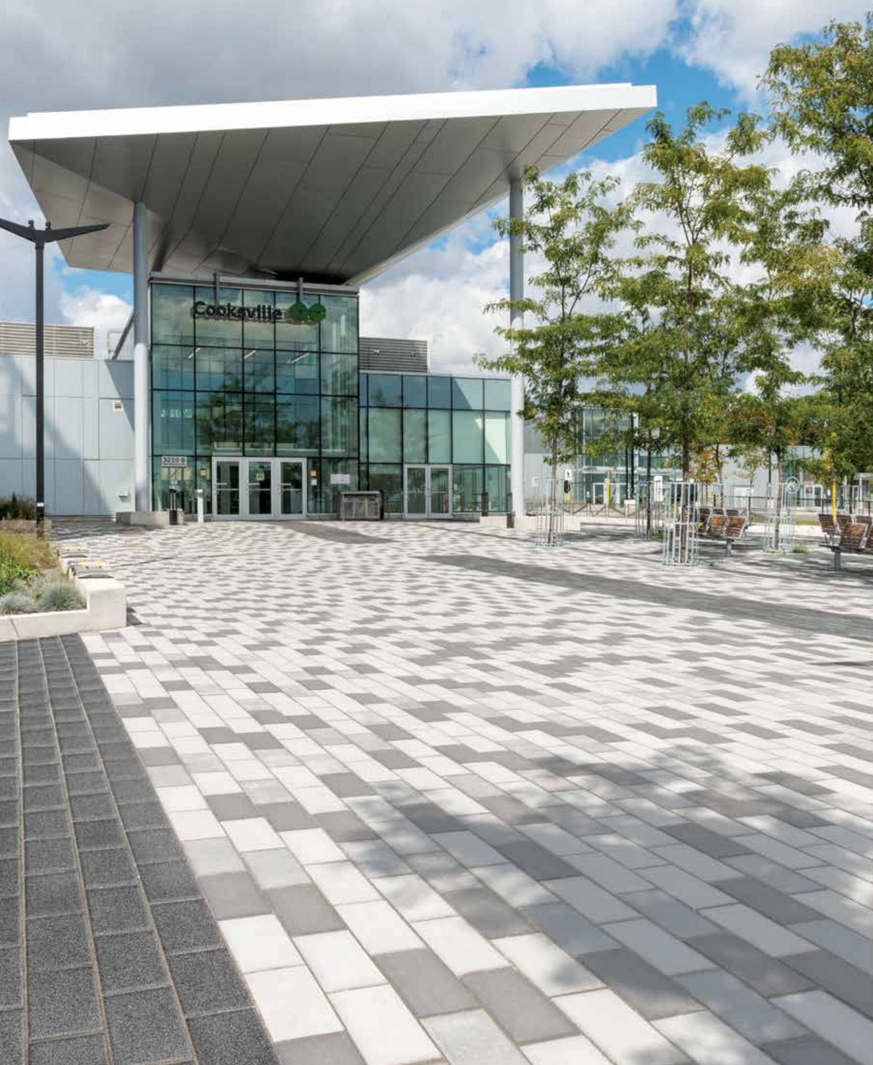
PROJECT: Cooksville GO Station, Mississauga, ON DESIGN: Brodies & Associates. PRODUCT: 7 x 14" with Smooth Premier finish in Granite Fusion, Midnight Charcoal and Opal Blend, and Series® finish in Black Granite.
