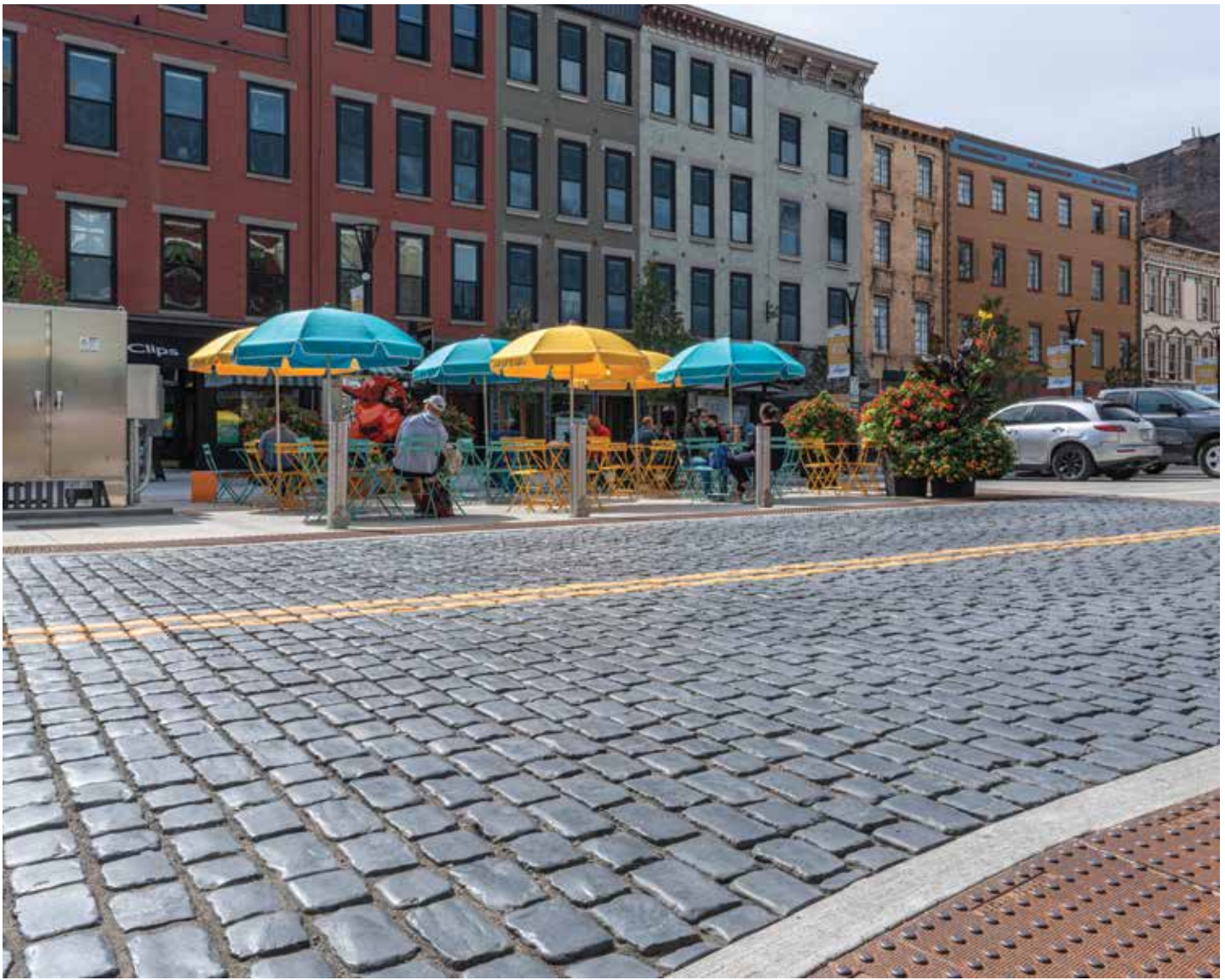
PROJECT: Court Street Plaza, Cincinnati, OH. DESIGN: Human Nature Inc. PRODUCT: Courtstone® in Belgian Blue.
