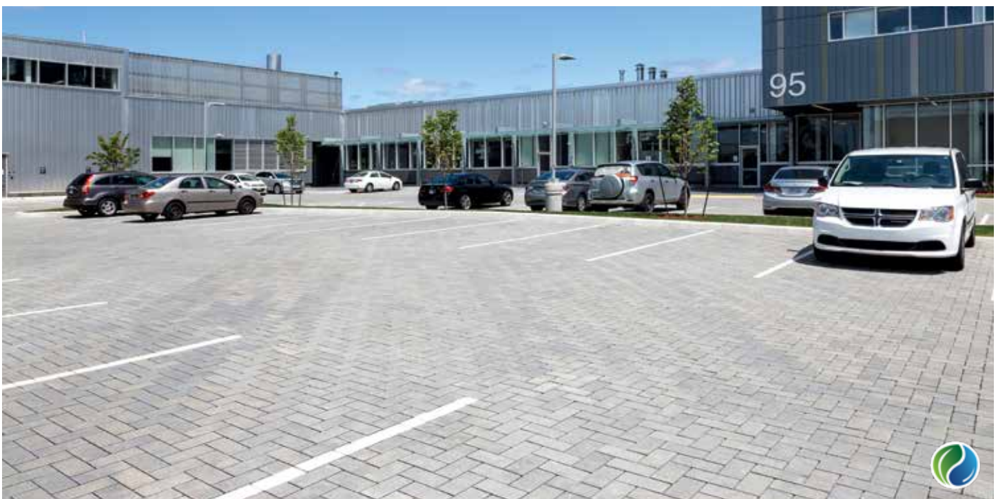
PROJECT: MTO Centre of Excellence, North York, ON. DESIGN: WSP Thornhill. PRODUCT: 5 x 10" Permeable with Il Campo® finish in Santa Fe.
