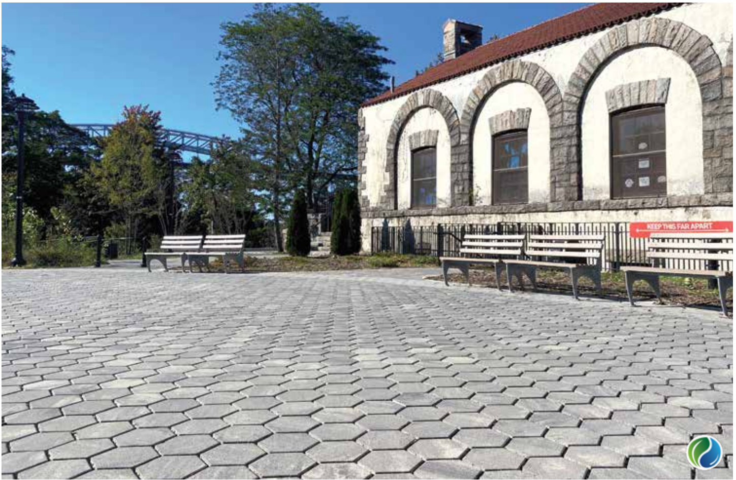
PROJECT: Faber Park, Staten Island, NY. DESIGN: Mark K. Morrison Landscape Architecture. PRODUCT: Hex / City Park Paver™ - Permeable with Smooth Premier finish in Steel Mountain.
