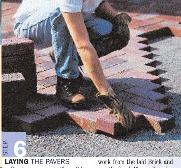
a. Start at a corner — if possible, one that includes a fixed edge, such as a wall, curb, or existing sidewalk. Set one run of Pavers on the Sand, from the corner along two adjacent borders. They should fit with about 1/16" — 1/8" gap between each Brick. As you go, be sure to
