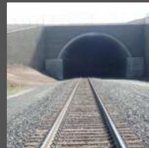
BNSF Tunnel Spokane, WA
