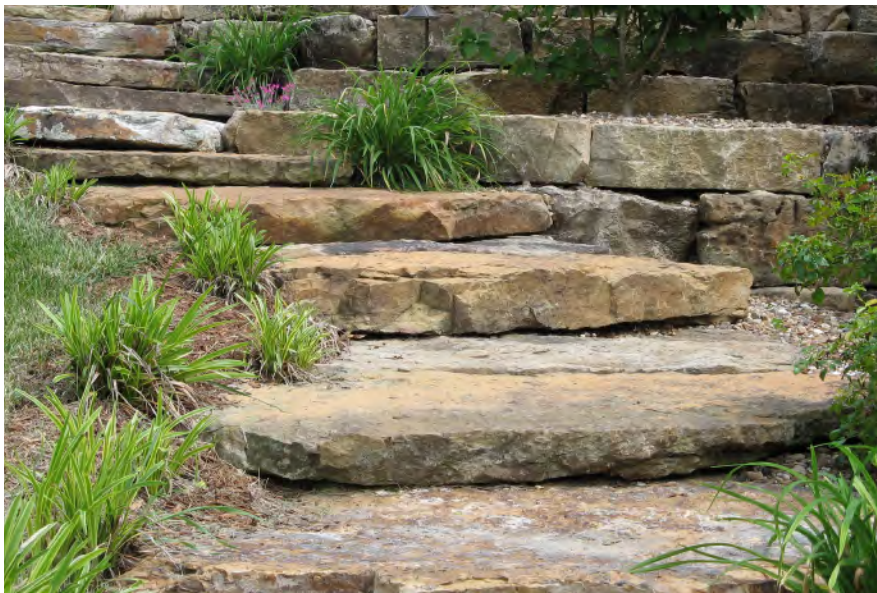
Weathered Sandstone Irregular Steps
