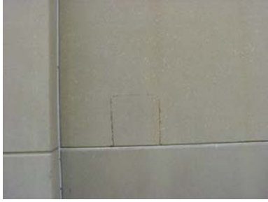
Fig 1. PWS applied to a 2x2 area on wall previous day
